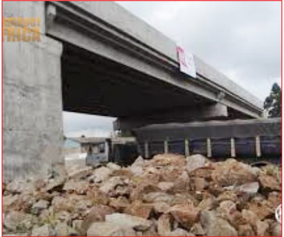
Construction of Flyover at Waiyaki – Nairobi Kenya
